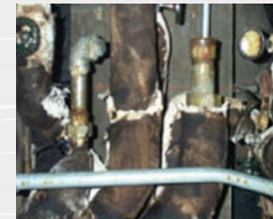
Asbestos Containing Materials (ACM) Inspection
